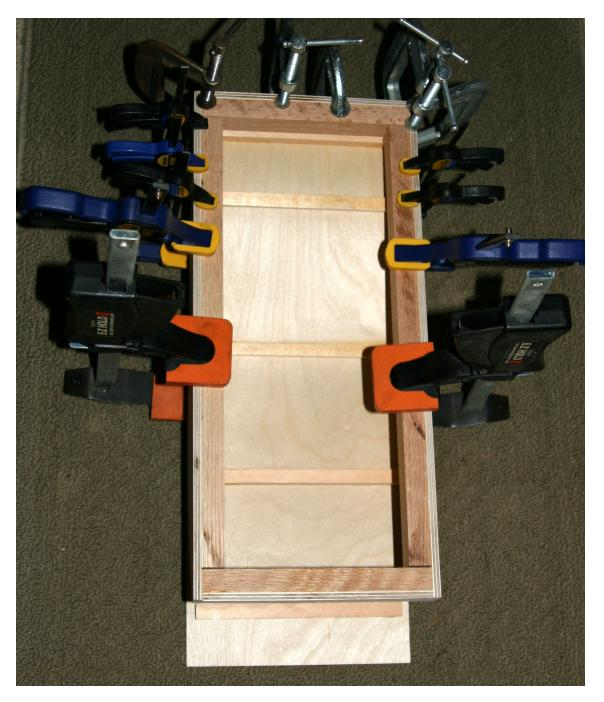
As soon the glue set on the bottom I put some scraps of fiberglass and resin along the inside seam to reinforce the joint. The sides have very little surface area for the glue to hold and I felt that that joint needed reinforcement before any other work could be done on the boat.
